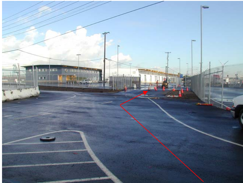
Entrance to Facility yard
